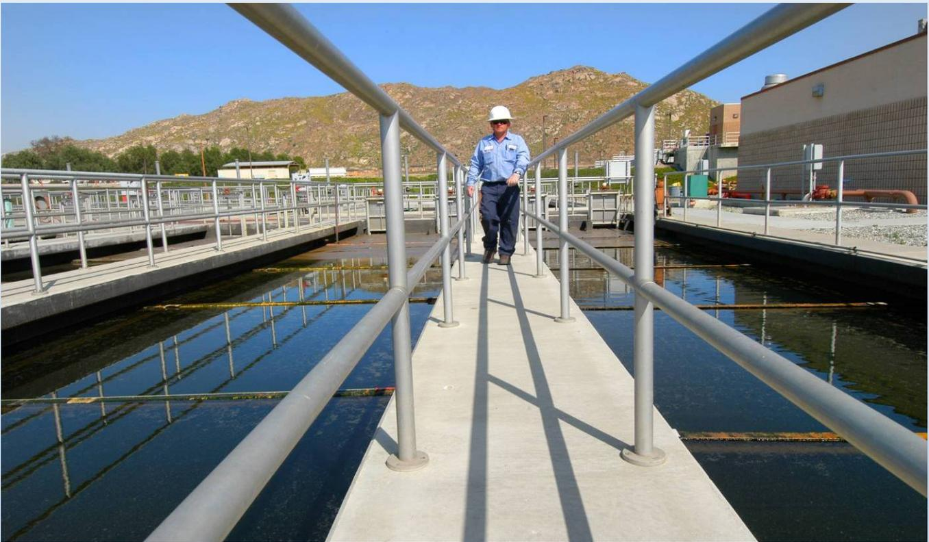
*Employee Bill Walker, Moreno Valley Water Reclamations Operator Grade III, performing a walk inspection in the plant 's #1 secondary clarifier which is an inactive environment where solids are settled out prior to tertiary treatment*
